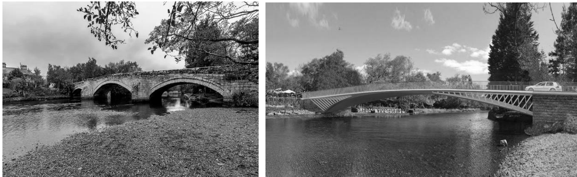
Figure 3. The 16 th century Pooley Bridge (left) & 'new' Pooley Bridge (right)
