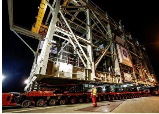
Figure 3. An example of an oil & gas module during the installation phase
