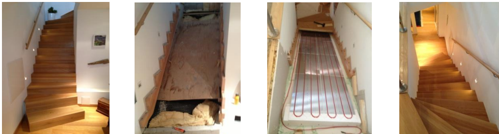
Figure 8. The different steps to make a cold stairway nice to walk in
