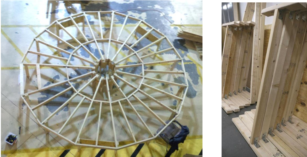
Figure 3. The platform assembled (note the office chair for scale) and disassembled into modular components. The flooring is removed to reveal the structure
